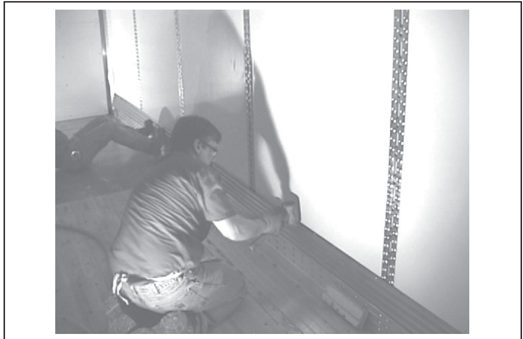
Figure 2-11, Reinstalling the Scuff Liner
