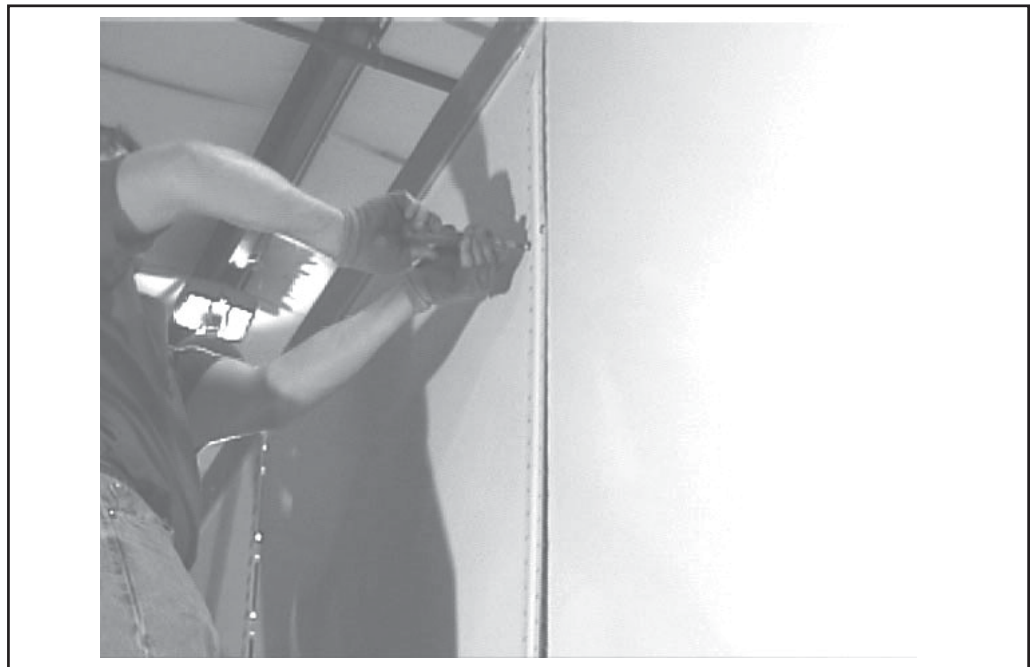
Figure 2-8, Installing Temporary Tack Bolts in the Vertical Seams
