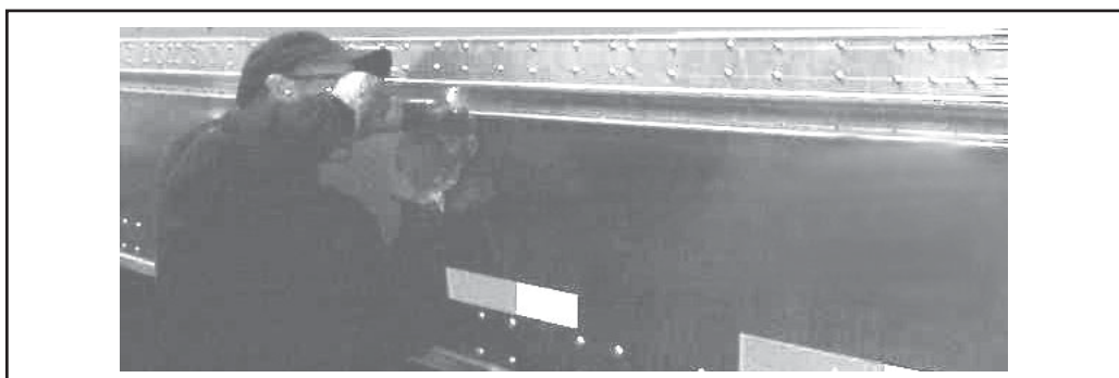
Figure 3-17, Bucking Rivets in Exterior Extrusion
