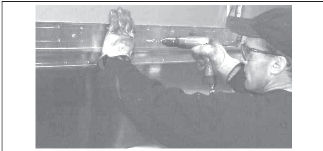
Figure 3-16, Drilling Through Replacement Panel
