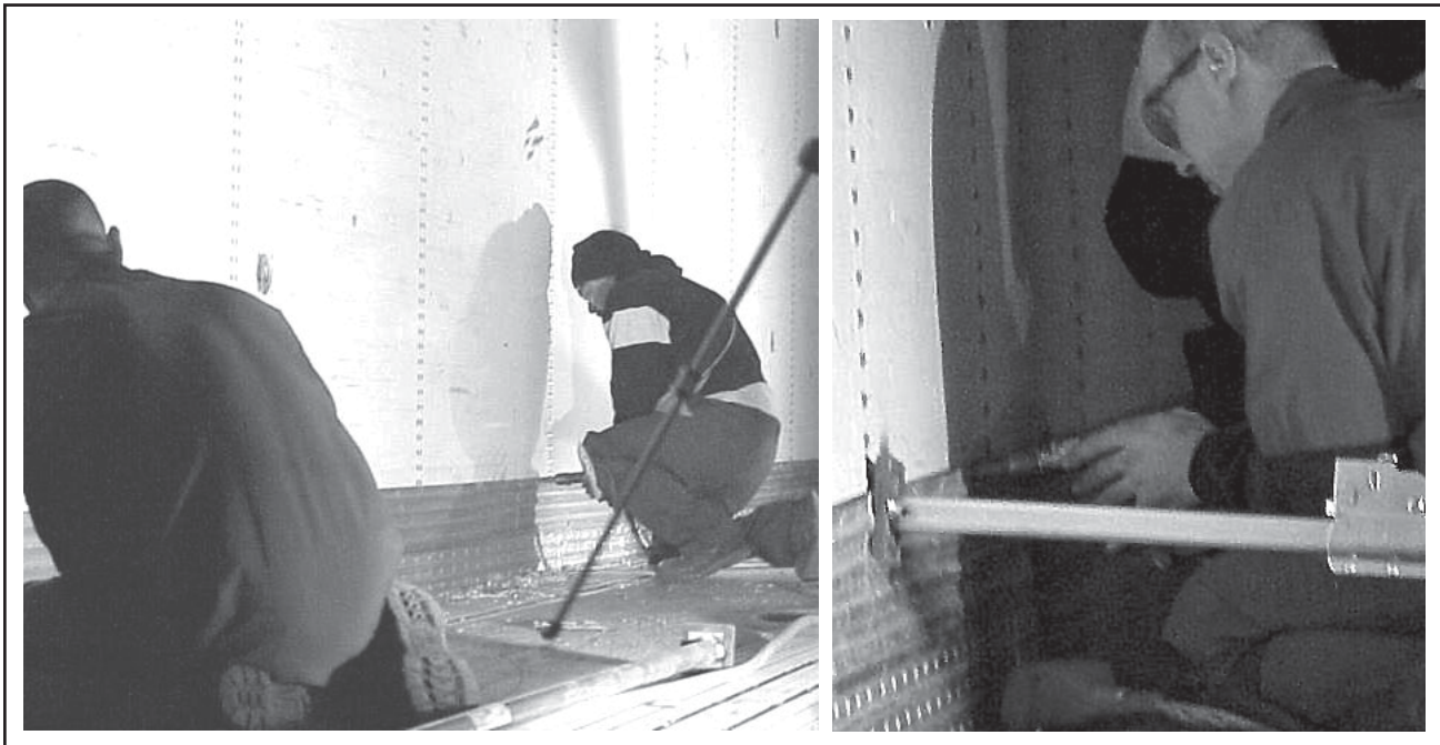
Figure 1-10, Reinstalling the Scuff Liner
