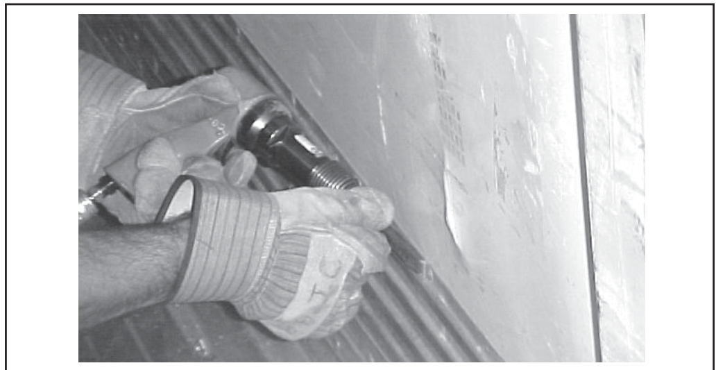
Figure 1-2, Removing Scuff Liner
