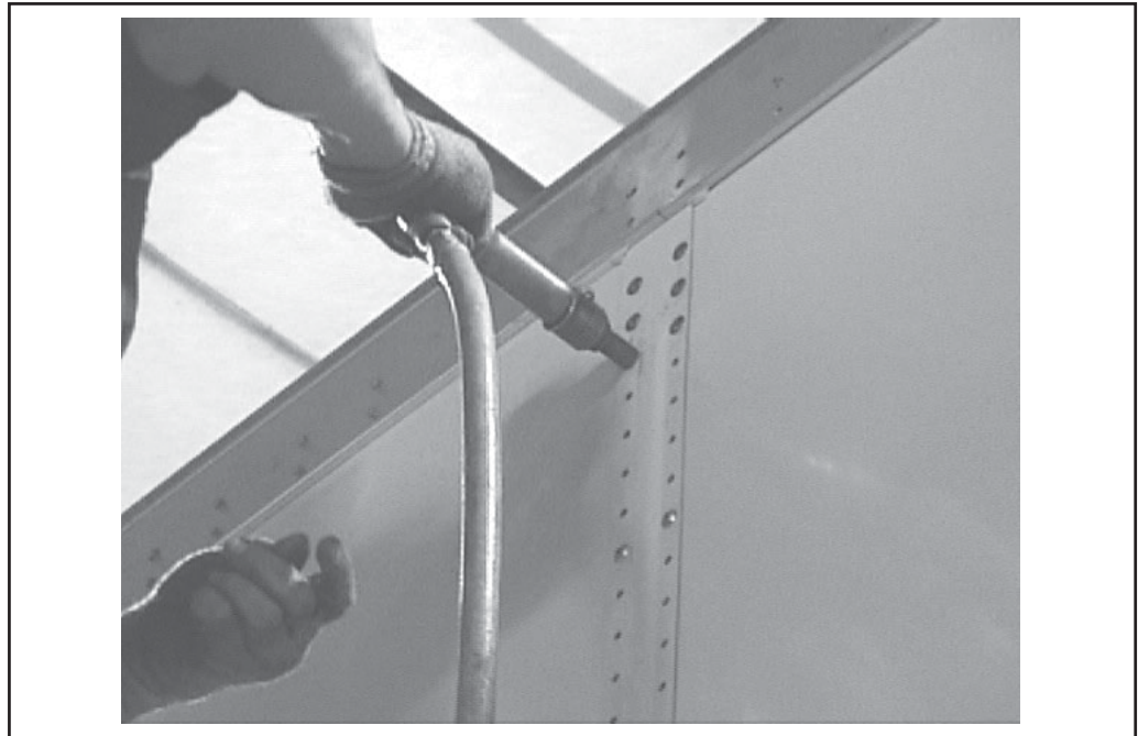
Figure 3-14, Installing Permanent Rivets Between the Tack Bolts from the Top Down
