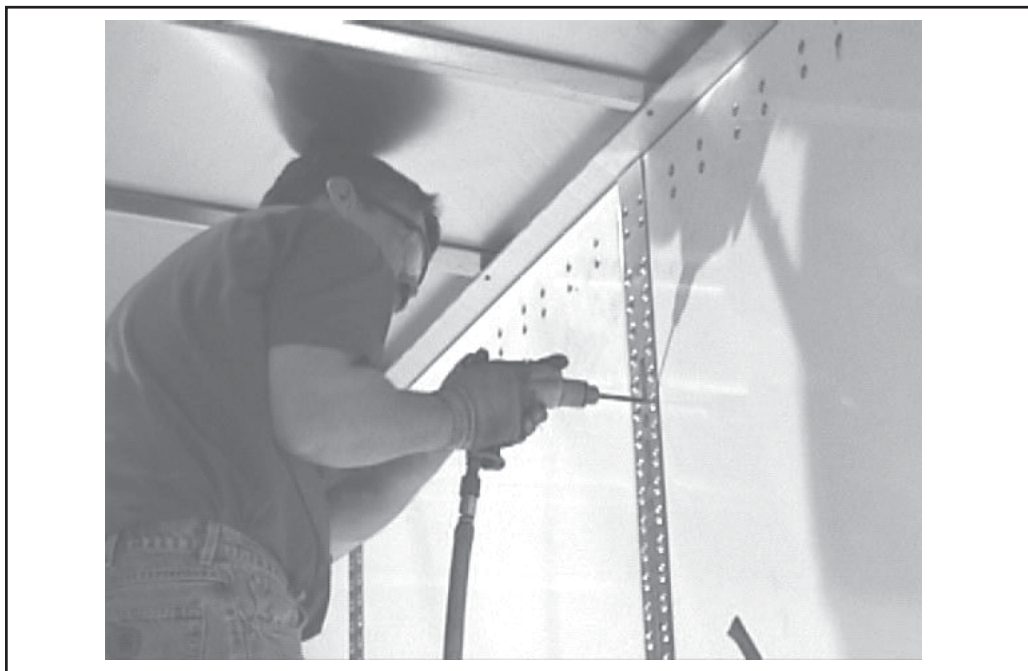
Figure 3-2, Drilling Out the Seam Rivets
