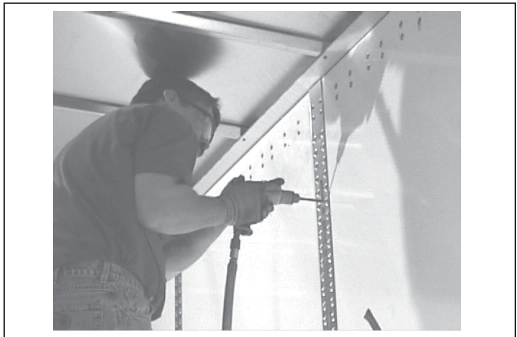
Figure 2-3, Removing the Vertical Seam Rivets
