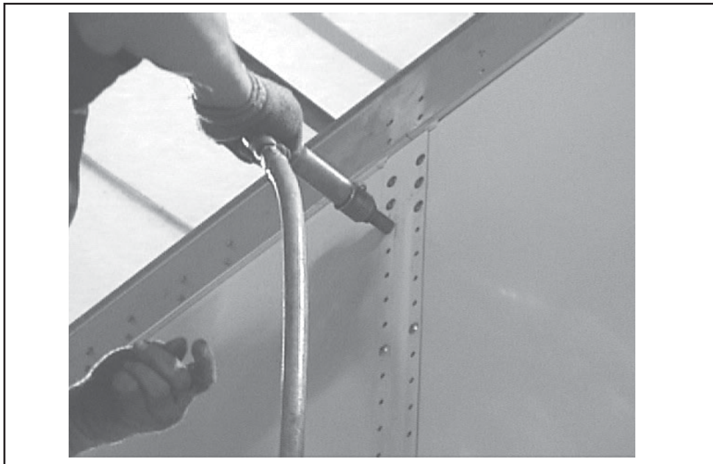
Figure 2-9, Riveting the New Vertical Seam Between Tacks
