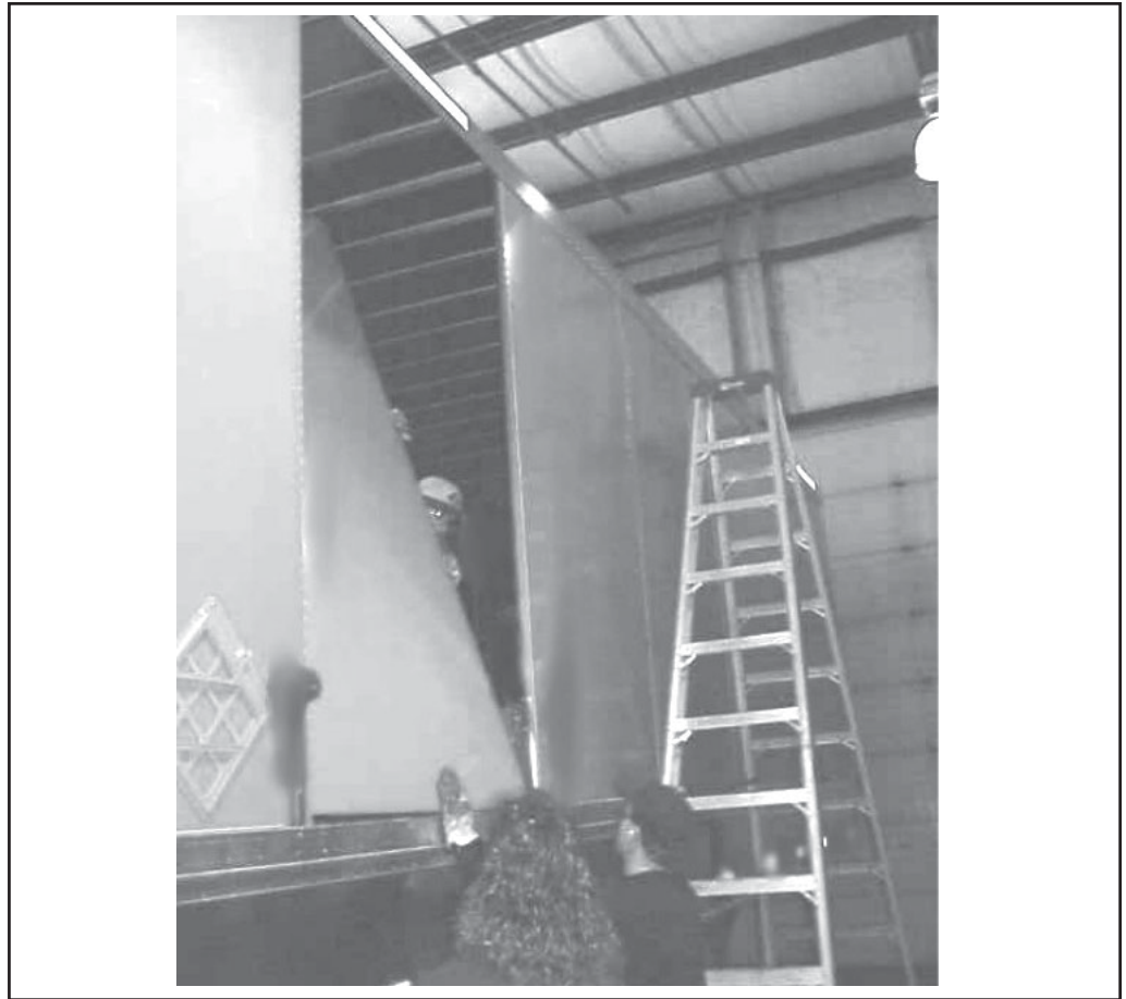
Figure 3-8, Lifting and Setting the New Panel Behind the HD
