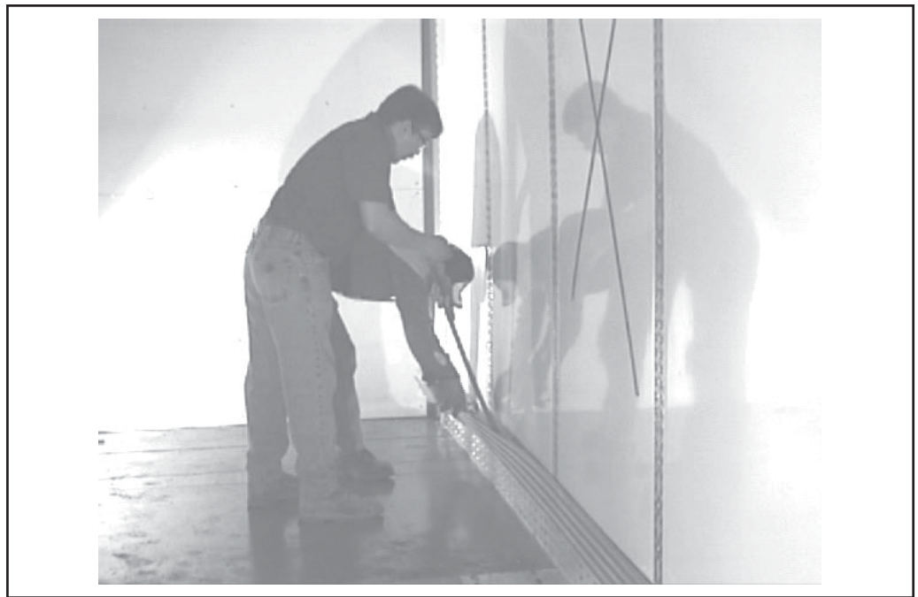
Figure 2-1, Removing the Scuff Liner
