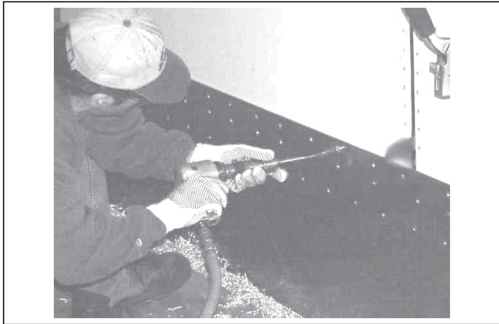
Figure 3-4, Punching Out the Base Rail Rivets
