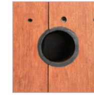
Pipe Pocket in Floor
